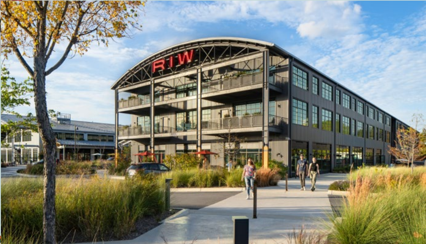
RALEIGH IRON WORKS / Raleigh, NC
