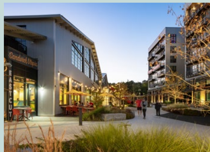
RALEIGH IRON WORKS / Raleigh, NC
